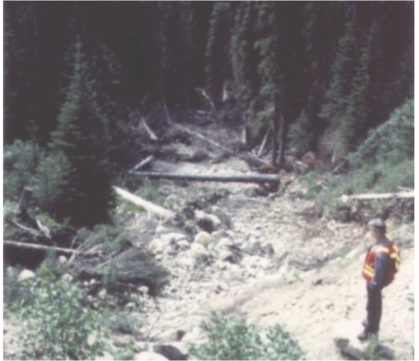
Figure 13. Road construction on steep, unstable glaciofluvial deposits in Kiwa Creek results in debris flows and soil erosion.
